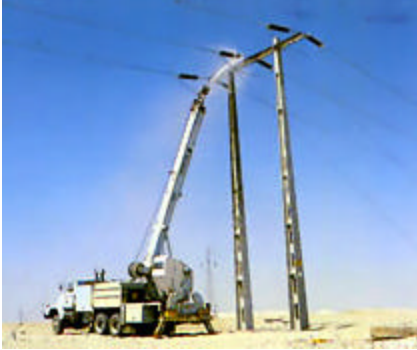
Figure 1: Live line insulator washing of a transmission line.
